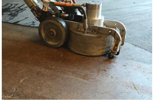
A high-pressure water-jet will quickly clean and prep a concrete surface with surprisingly little water, with the surface returning to its original dry state in a matter of minutes.
