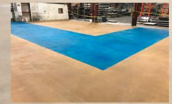
Endurable Polymer Pavement with sand broadcast and stain
