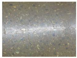
When aggregate is exposed, you need a grout that is close to the color of the cement paste. Seen here, the grout in the light reflection area is not yet as high gloss as the rest of the floor. When polished it is almost impossible to see if the color is selected properly.
