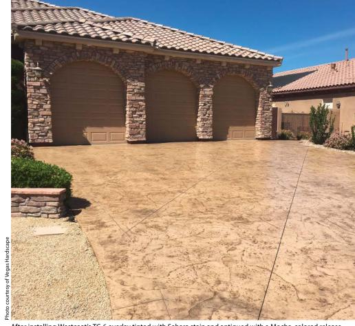
After installing Westcoat's TC-6 overlay tinted with Sahara stain and antiqued with a Mocha-colored release, contractor Mike McAnulty stamped this driveway with an Old Granite pattern from Proline. It was then sealed with Arizona Polymer's Poly 250.
