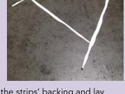
the grout coat has cured, peel off the strips' backing and lay them out end-to-end, taking time to reposition as needed and inspecting for consistency prior to applying the texture coat.
