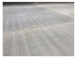
When the glue or mastic is abated, the finish is usually shot blasted, removing the entire paste cap of the slab.
