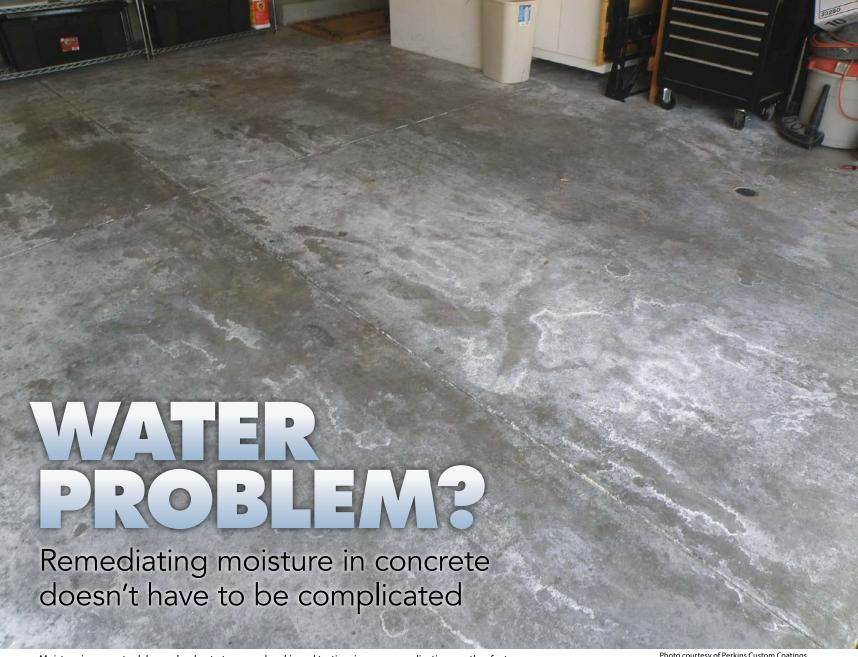
Moisture in concrete slabs can be due to topography, skipped testing, improper application or other factors. Seen here is severe blooming efflorescence, one of the unsightly results of excess moisture.
