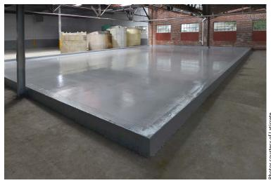
One coat of Drytek's two-part epoxy coating can effectively control the moisture vapor emission rate from new or existing concrete slabs.
