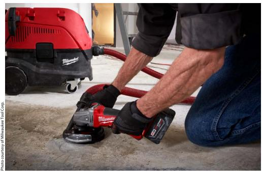
Battery life depends on how frequently and consistently a tool is used on the job site. Grinders, which typically are used continuously for hours, have proven to be a challenge.
