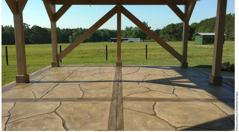
Jeremy Bayliss's Busted to Beautiful system using Elite Crete products turns cracks into stone by cutting, carving and resurfacing the cracked surface. This process is becoming very popular for his company and many other installers around the country have been trying to learn the process. For this project in Slocomb, Alabama, Bayliss turned existing cracks into a wood and stone design.
