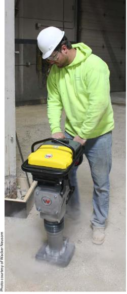
A battery-powered rammer allows for compaction without a power cord or emissions.
