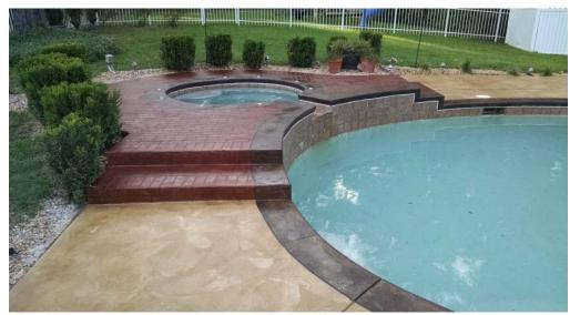
This pool and spa features a combination of a brick and tile design alongside a plain textured area for visual relief. Crack repair on this job was done using concrete staples. The job was hand-troweled and hand-stained.
