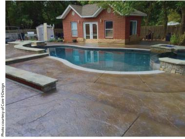
After stamping this pool deck in Broken Arrow, Oklahoma, and staining it with a series of grays and walnuts, Andy Jones applied a proprietary dry pigment mix that gives the surface color-changing qualities. To tie it all together, he then added glow resin around the pool inside control joints and decorative cuts.
