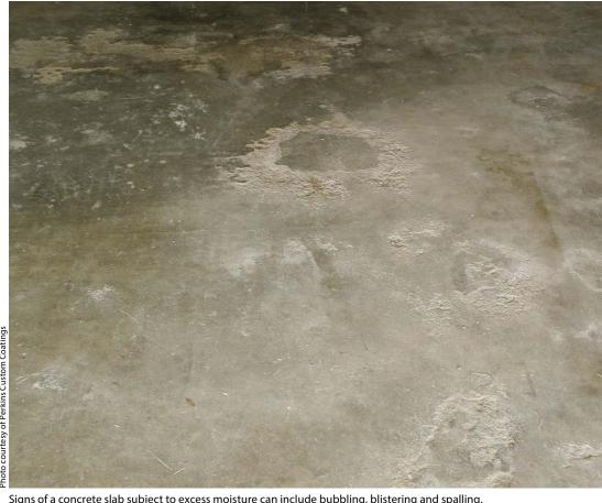
Signs of a concrete slab subject to excess moisture can include bubbling, blistering and spalling.
