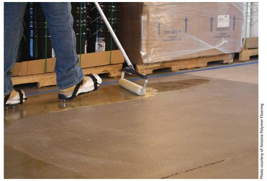
Applying an epoxy coating such as VaporSolve Ultra System from Arizona Polymer Flooring is a simple remediation to seal in moisture — whether you know if it's present or just suspect it.
