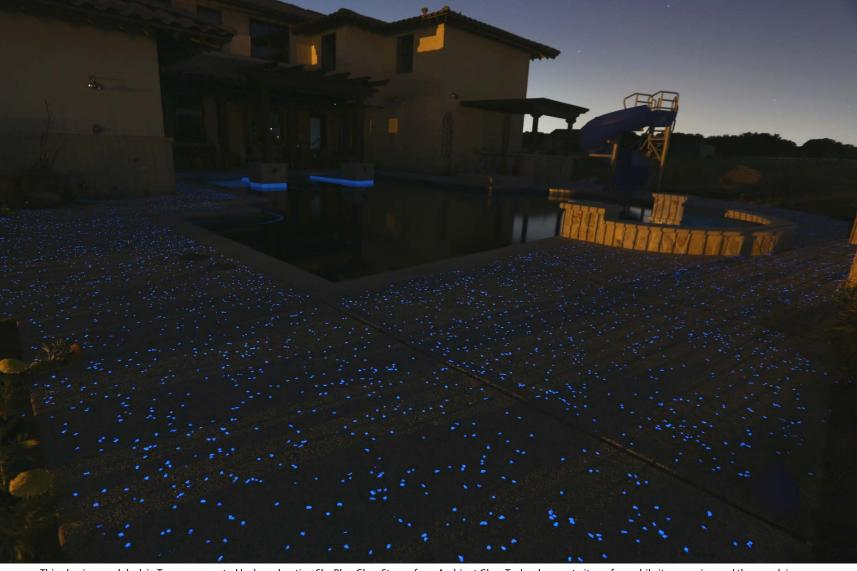
This glowing pool deck in Texas was created by broadcasting Sky Blue Glow Stones from Ambient Glow Technology onto its surface while it was curing and then applying a retarder. The surface was then finished with a light pressure wash. Below is what it looks like by day.
