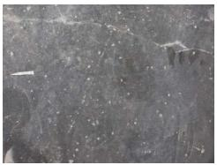
are several hundred thousand screw chips in this high-end floor. All the white dots in this photo are chips in the concrete surface. (See photo above.)
