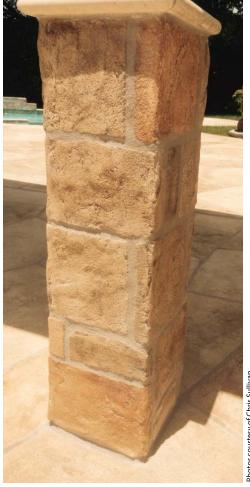
On vertical applications, a limestone overlay can be applied up to 3/4 inch thick.
