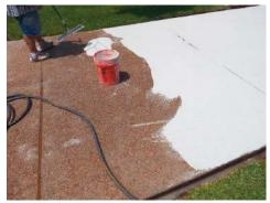
A scratch coat of limestone overlay is applied over pea gravel-exposed aggregate.
