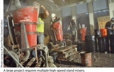
Lastly, don't forget to match the blade shape with the mixing container. Mixing blades with a taper or rounded tip don't work well with flat-bottomed mixing containers. Ryan recommends tapered mixing drums, without corners, to avoid material collecting, which can result in inconsistent mixes and dry clumps.
