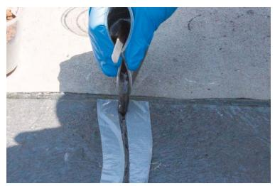
Especially with epoxy-based systems, some products can leave a stain on the adjacent concrete. In those cases, it pays to apply a mask before doing the work.
