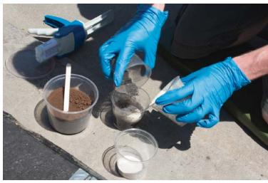
Depending on the manufacturer, fillers and sealants are offered in a wide range of standard colors. Custom colors still call for a good eye and a little handwork.
