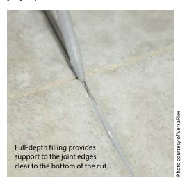
control joints and construction joints.
