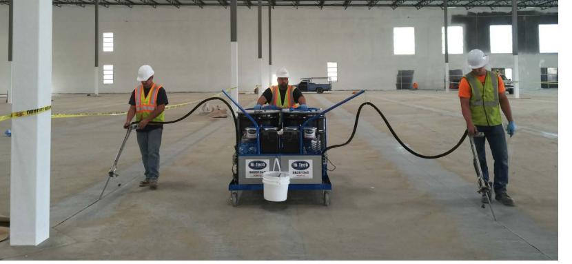
A big job can require big equipment. This large pump, designed especially by Hi-Tech Systems, allows two workers to dispense polyurea at the same time. Photo courtesy of Hi-Tech Systems
