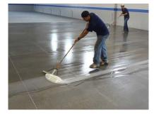
days after pouring new concrete. This reduces the waiting period between pouring, priming and finishing by as much as 18 days, saving valuable time while accelerating project timelines.
