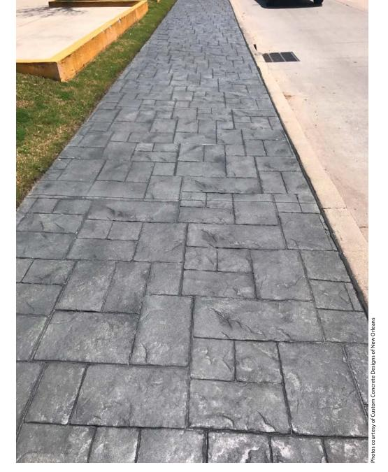
Hudgens cites a recent project in Louisiana as an example of the stain-and-seal system's application. Here, the aging green color of stamped sidewalks in a busy commercial district dictated a total do-over using a nonfilm-forming color system. Initially thinking he'd have to demolish the stamped surface, the owner was advised of the stain-seal alternative. The cost and time reduction were substantial, says contractor Steve Malone, owner of Custom Concrete Designs of New Orleans.
