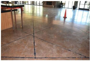
This floor was in such sorry shape the contractor couldn't tell the color of the caulking he was replacing. Once a black polyurea had been applied, the overfill was cut back (left) and the floor is ready to be ground and polished (right).
