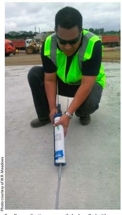
Smaller applications can easily be handled with a cartridge system of premixed product.
