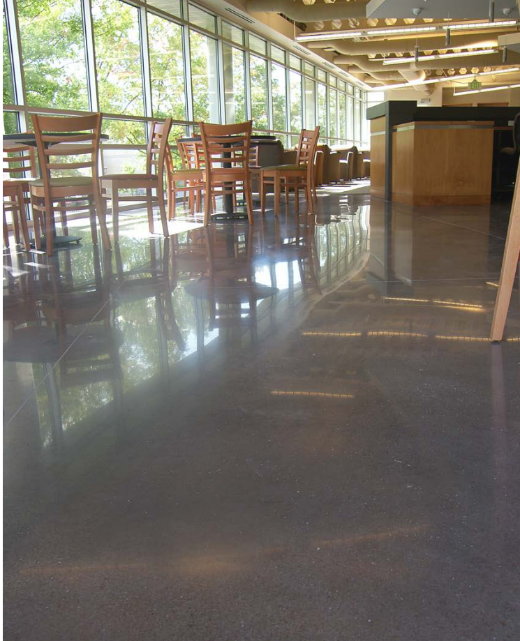
A mechanically polished floor that's done properly will have reflections that are crisp and clear.
