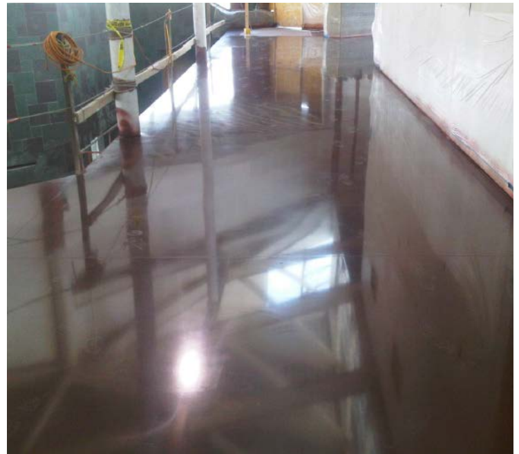
Lights will have reflections with "tails" on floors that are tainted by resin transfer.
