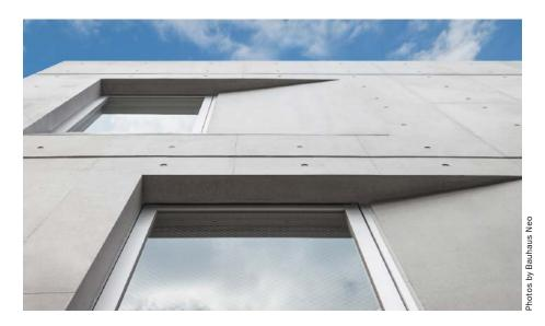
Its most striking feature is the window treatment. From inside, the windows appear sufficiently large, but on the outside the surface surrounding each one slopes in at an angle, creating a recessed "frame." Some of the sloped surfaces are covered with hot-dipped galvanized steel sheets.
