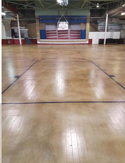
The gym's original wood floor had been replaced with a carpet court, which Bell and his crew pulled up to reveal a precast concrete base. After filling in all the cracks, they put down a scratch coat of Stone Edge Surfaces' Pro Bond before applying Pro Spray, "which gave us a wood grain look," Bell says.
