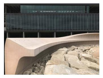
Installation required some creativity, innovation and tight planning. The precast panels were mounted on a cast-in-place kneel wall using both column-base connectors on the land side and splice sleeves on the lake side. This unique system, developed just for this project, allowed the contractor to bolt the panels in place without using an interim bracing system.
