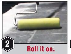
Roll or brush apply the biodegradable Deco-Peel liquid stripper over the blanket until saturated. Allow the liquid to dry (usually 2-4 hours).
