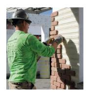
features brick seating for each row of brick. Once the first panel is level, you're good to go. No weeping system behind the panel or special tools are needed to install.
