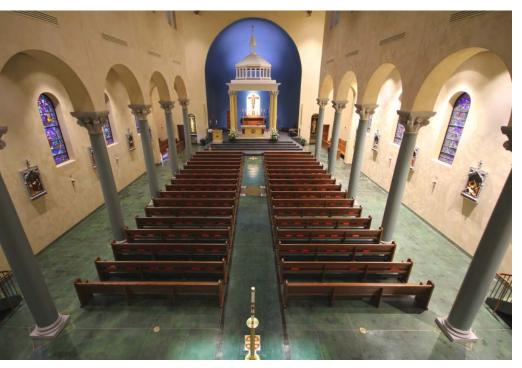
have ended up looking like a line right down the middle of the sanctuary, but Simpson used a misting spray in the seal coat to help the colors blend. She also used the spray to add highlights to other areas of the floor, unifying the overall effect.
