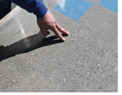
Hi-Tech Systems displayed how stealthy its Spall-TX3 could be. You can barely see where the polyurea concrete repair material was used on this surface as it literally makes the repaired area disappear. This rapid-set, 100 percent solids material is designed to rebuild and repair broken control joints and spalled concrete. On top of that, it's polishable. (\$) www.hitechpolyurea.com
