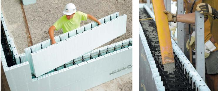
According to ICF manufacturers, insulated concrete form construction combines several wall-assembly components in one unit: Concrete, steel reinforcement, insulation, air barrier and vapor barrier.
