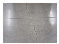
Crack chased and filled
